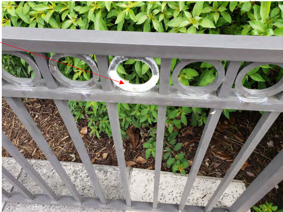
Decorative rings are heavily corroded and will need to be stripped.
