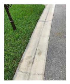
**Description:** Moderate fractures in valley gutter curb.
