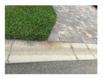
**Description:** Moderate fractures in valley gutter curb.
