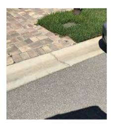
**Description:** Moderate fracture in valley gutter curb.
