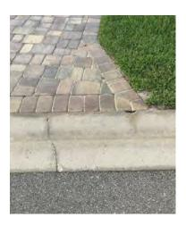
**Description:**Multiple moderate fractures in valley gutter curb with missing concrete.
