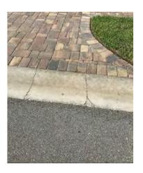
**Description:** Moderate fractures in valley gutter curb.
