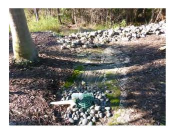
**Description:** Berm is eroded and potentially breached.
