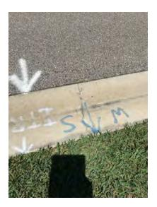
**Description:** Moderate fracture in valley gutter curb.
