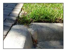
**Description:** Type "F" curb is fractured with missing concrete
