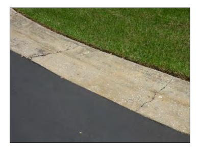
**Description:** Moderate fractures in valley gutter curb.
