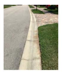
**Description:** Moderate fracture in valley gutter curb.
