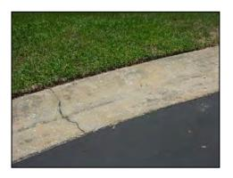
**Description:** Moderate fracture in valley gutter curb.
