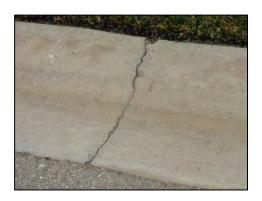
**Description:** Moderate fracture in valley gutter curb.
