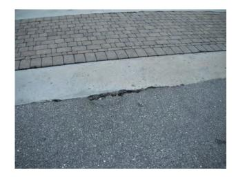
**Description:** Pavement settling at ribbon curb.
