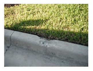
**Description:** Type "F" curb broken with missing concrete pieces.
