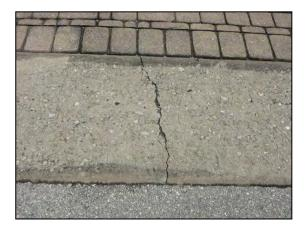
**Description:** Moderate fracture in ribbon curb at crosswalk.
