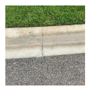
**Description:** Moderate fracture in valley gutter curb.
