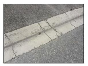
**Description:** Multiple fractures in valley gutter curb.
