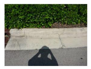
**Description:** Moderate fractures in type "F" curb adjacent to inlet.
